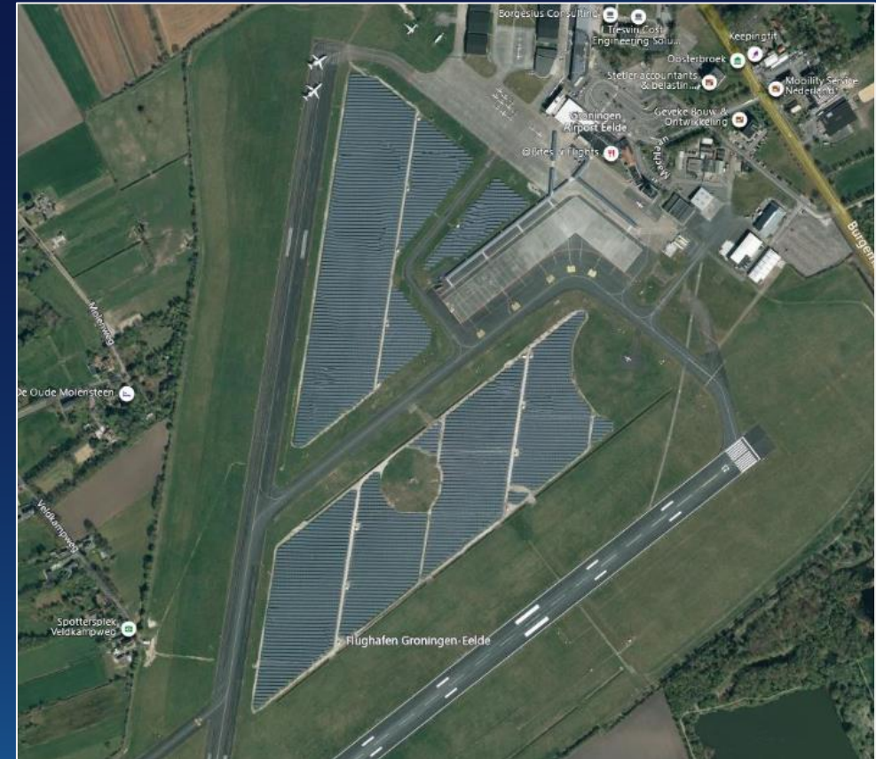
Groningen Airport, The Netherlands with a 22MW PV farm (north/south RWY INOP)
